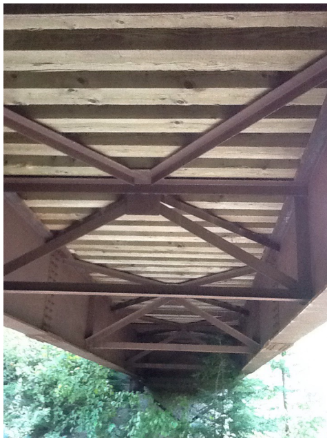
Underside of bridge
