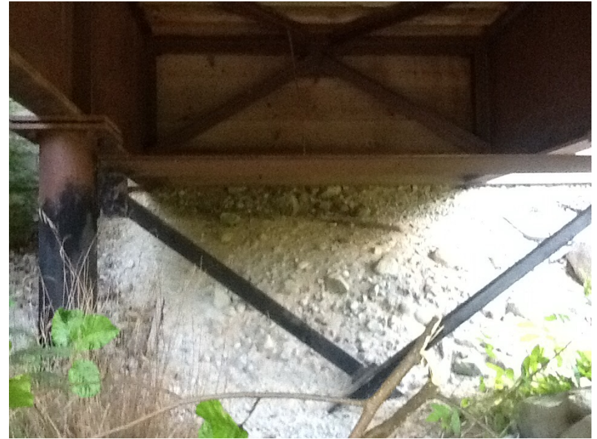
Left Bank Abutment when facing downstream
