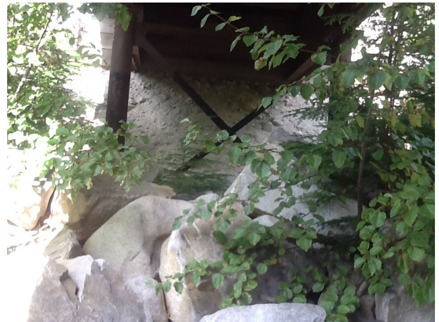
Right Bank Abutment when facing downstream
