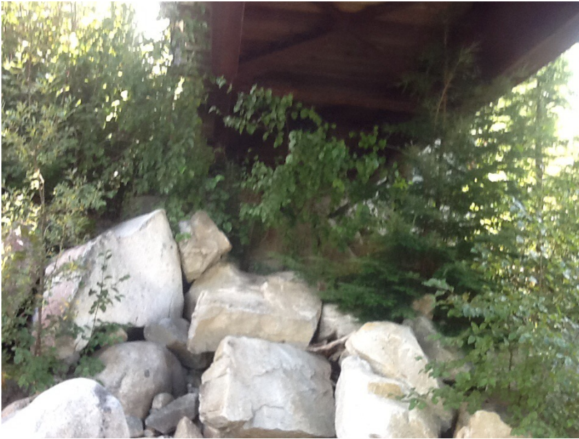
Left Bank Abutment when facing downstream
